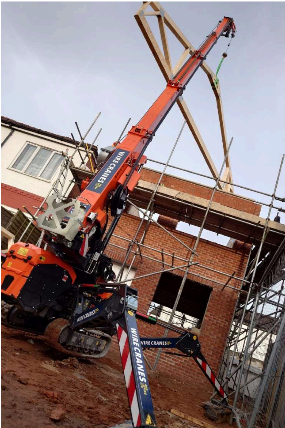
One of the spiders at work aiding in the construction of a house
